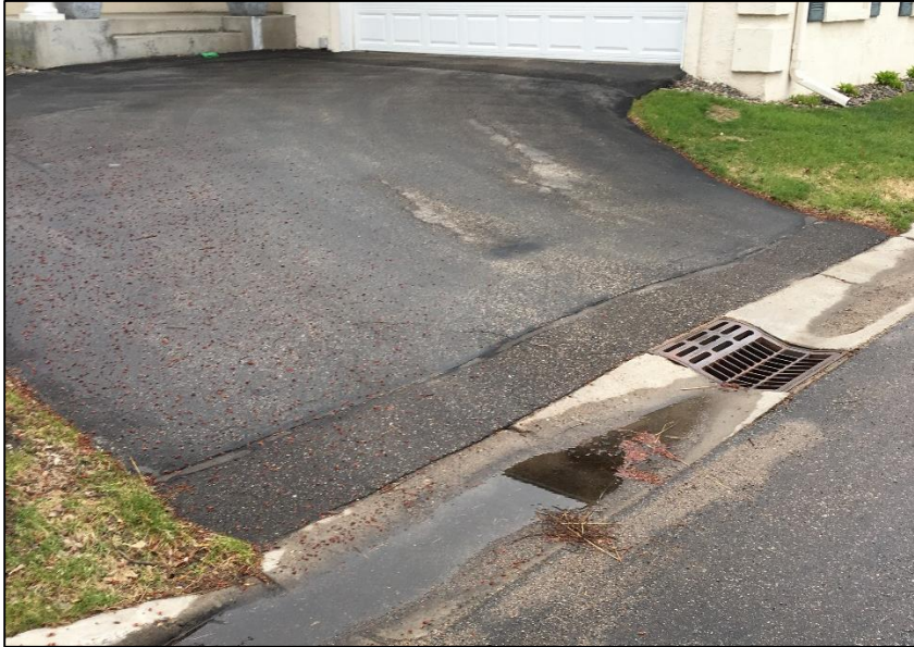
Photo 7. Patching at Curb Line and Garage Slab
